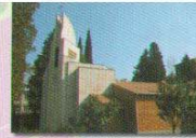
7 German Lutheran Church. 1995-97. Arch: G. Metreveli, U. Grefi Location: Terenti Graneli St.
