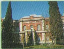
1 Silk Station Arch: A. Szymkiewicz Location: 6 G. Tsabadze St.
