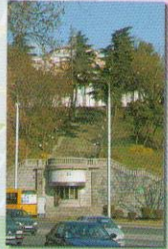
3 Tbilisi Circus Arch: V. Urushadze, N. Neprintsev, S. Satuntsi. (1940). The Rotunda is situated on the hill and can be seen from all the sides. It enters into the composition by means of the long stairway. Location: 1 Gmiria Square
