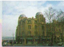
7 Melik Azariants's apartment building (1912-1915) Arch: Nikoloz Obolonski. Location: 37 Rustaveli Ave.
