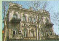
1 Apartment House The Facade - Renaissance motives. Arch: unknown Location: 103 Marjanishvili St.
